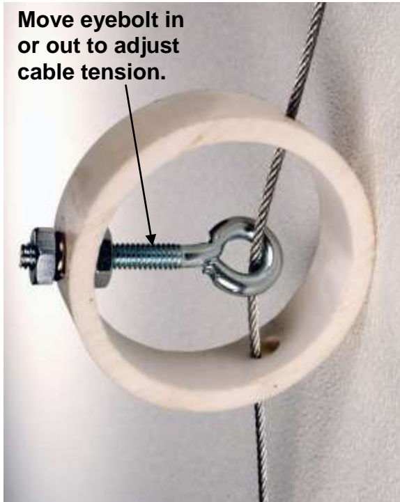
Photo # 5.31 (Cable Adjuster Assembly)
